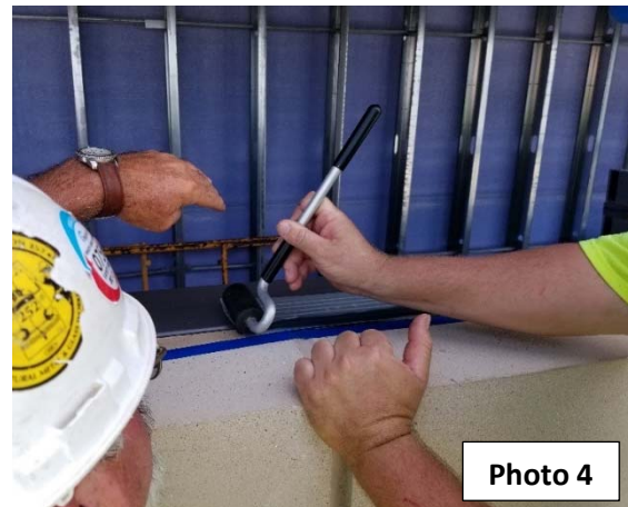
Wetting out adhesive with roller.
